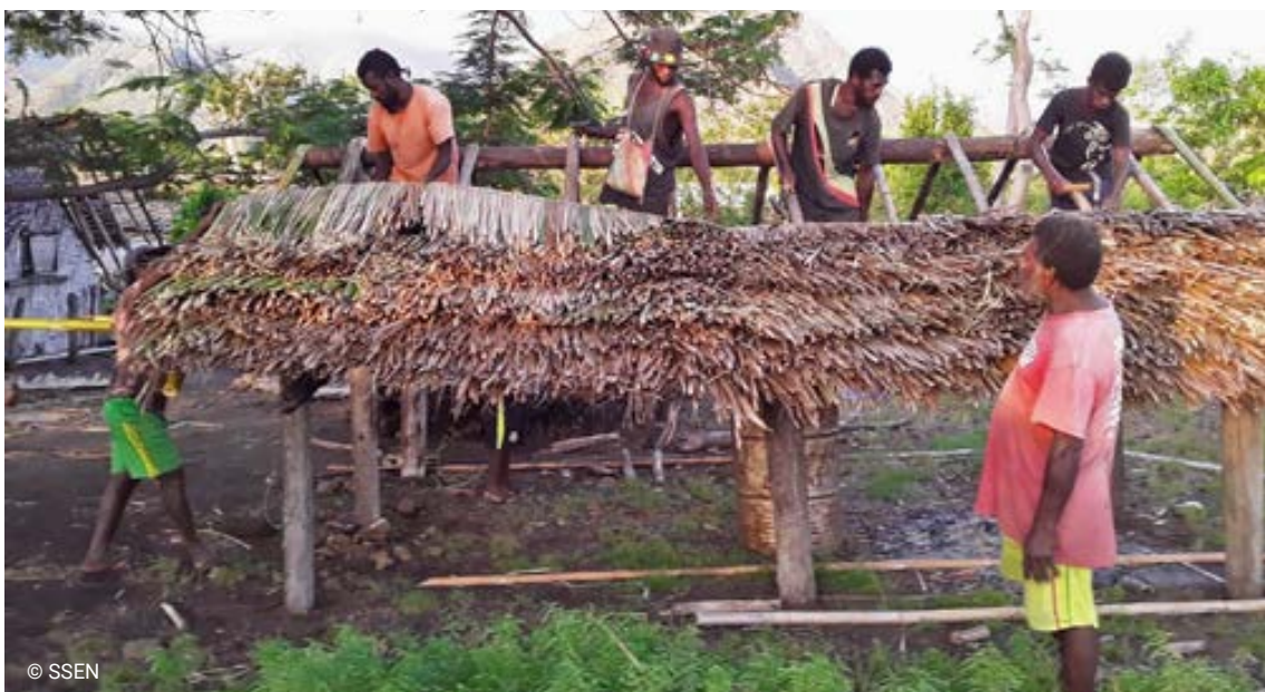
Community members construct a hurricane house.
