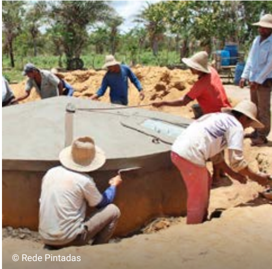
Production of water tanks to conserve precious fresh water and reduce evaporation in a heavily drought-affected climate.
