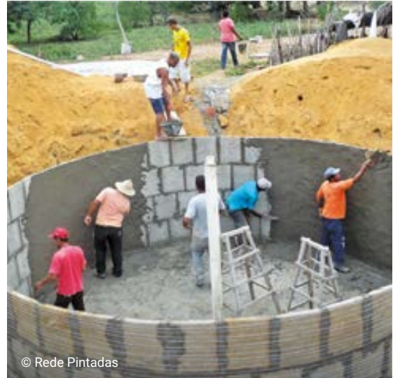
Production of water tanks to conserve precious fresh water and reduce evaporation in a heavily drought-affected climate.
