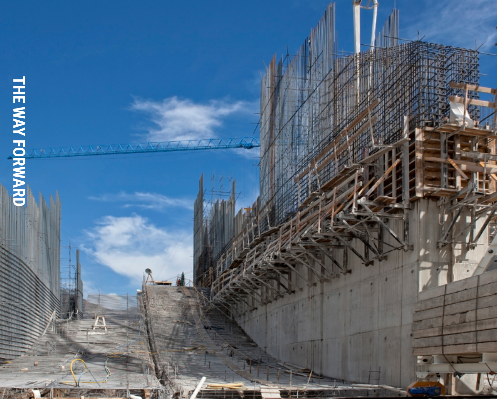
Hydroelectric dam construction. Picture: iStock
